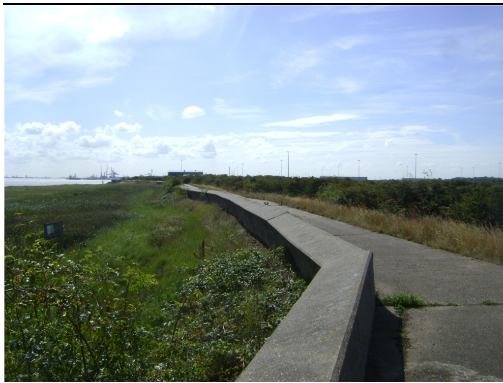
Figure 6.10 Estuary Flood Defences at Site
