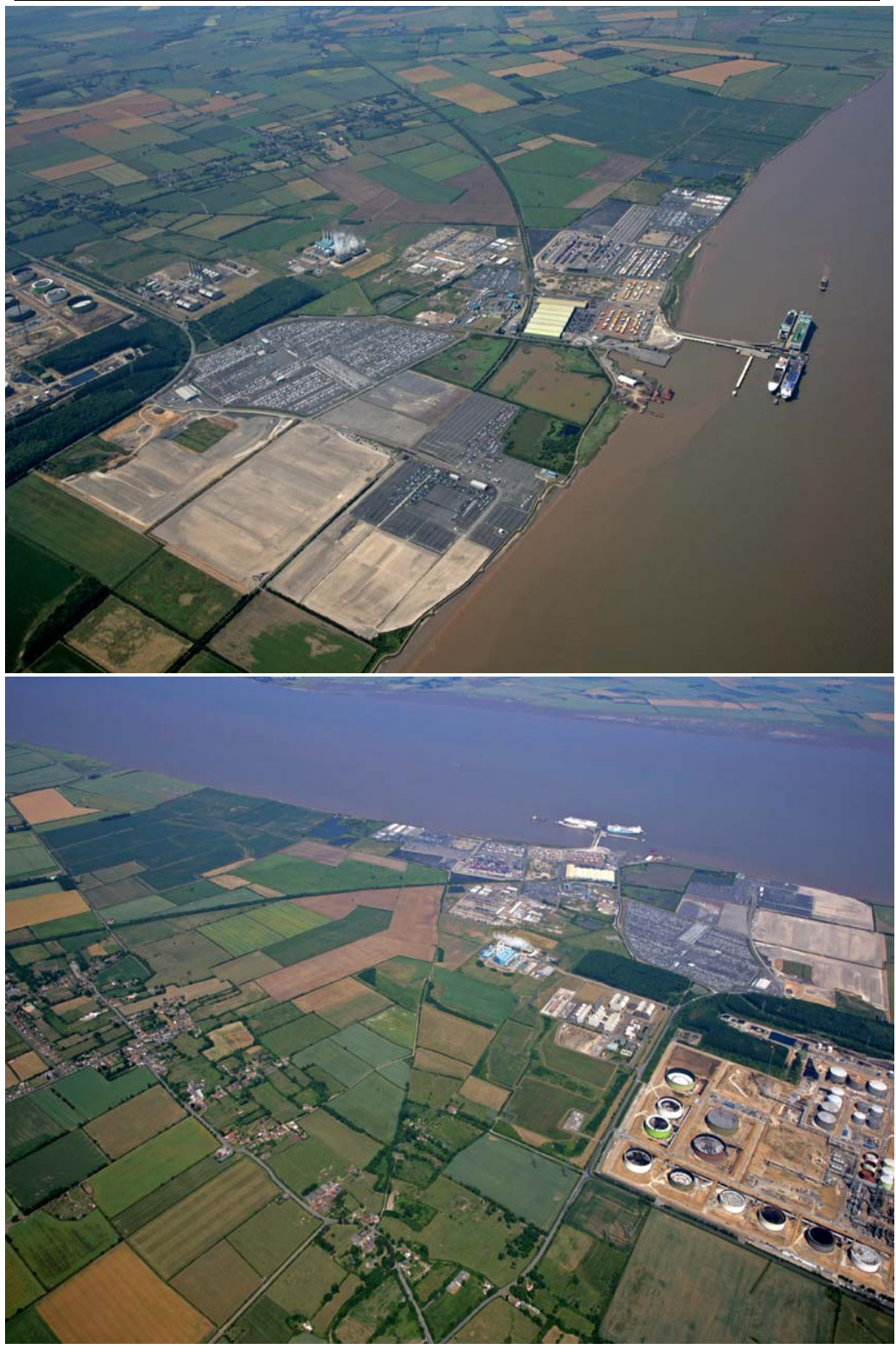
Figure 3.3 Existing Site Characteristics
